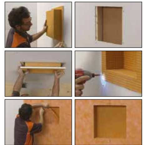
Installation in drywall
